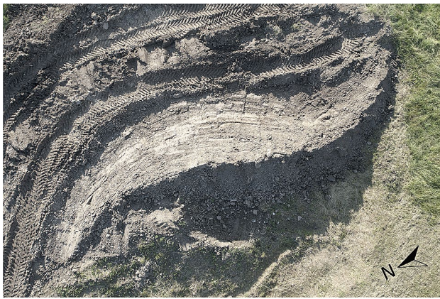
Fig. 13 A top view of the finished embankment prototype shows the curved design and the smooth surface finish
