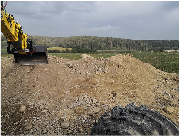
Fig. 19 The image shows the final state of the two-faced embankment experiment. An overall smooth surface finish with a clear and straight corner was achieved
