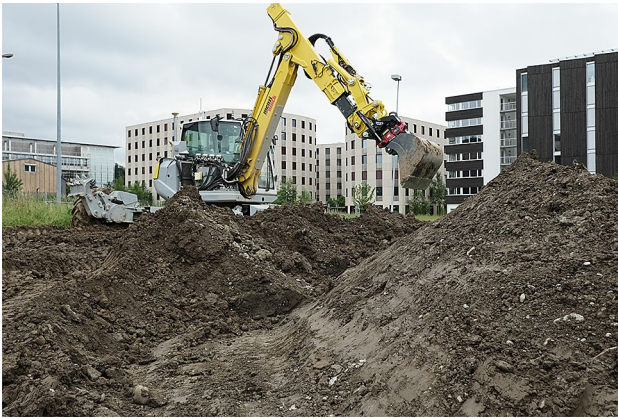
Fig. 1 The autonomous walking excavator HEAP can excavate free-form shapes with high accuracy. The image shows the s-curved embankment's progress with the finished surface in the foreground and the unfinished pile to excavate behind it
